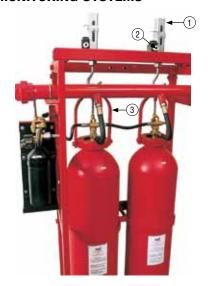
This device is used to automatically monitor the contents of the CO2 cylinder. When the CO2 gas falls the indicator on the device will show that it is empty and an optional Micro-switch can be installed to send a signal to the control panel. This is the most effective method of monitoring the CO2 gas in the cylinders.
